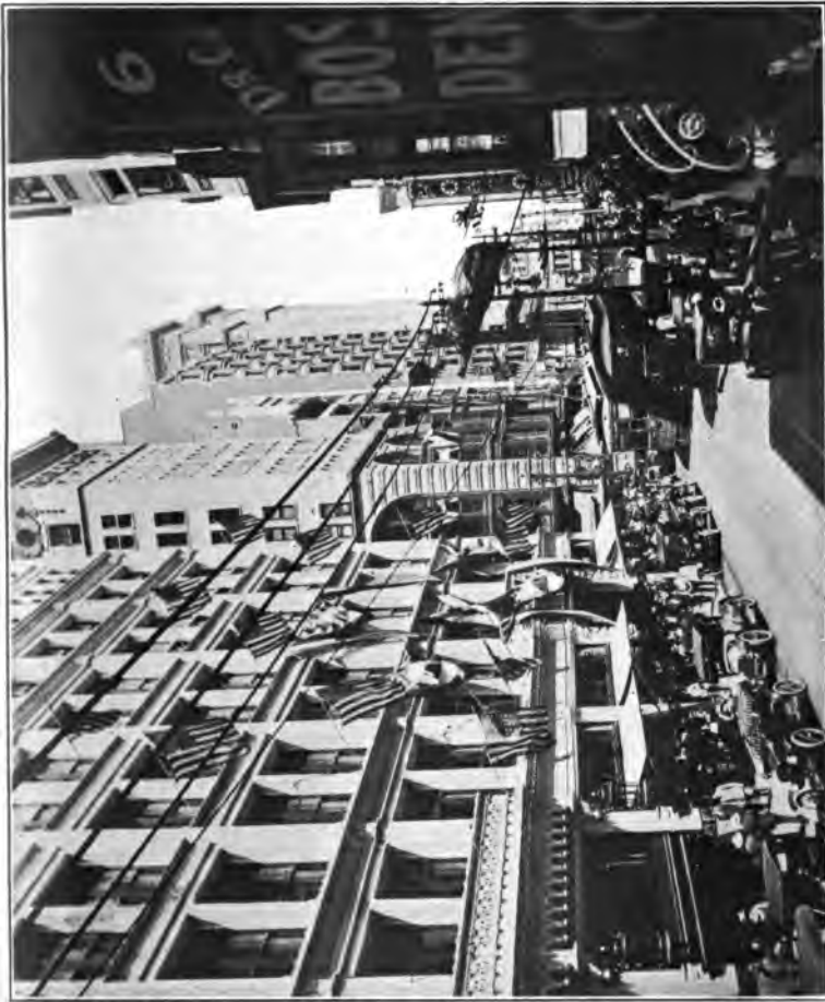
Illustration No. 3. —As St. Louis grew west from Fourth street a width of 60 feet in place of 30 feet was adopted for most streets. This view shows Olive street at Seventh. The complete inadequacy of a 60 foot street containing a trolley line as a traffic thoroughfare is well illustrated. There is room for but one automobile between car and curb, and this space is usually occupied by standing vehicles.
